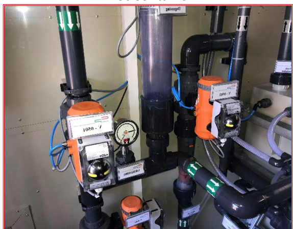
Control Valves and Degassing Chamber
